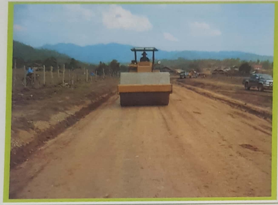
Figure No. 6 ROAD COMPACTION
