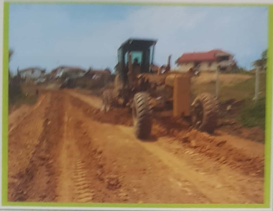
FIGURE NO. 4 STAB-TECK IN THE TREATMENT AREA
