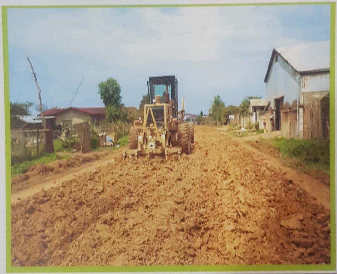
Figure No. 3 STAB-TECK MIX ON THE ROAD
